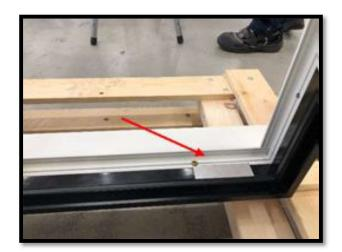
The position of the glass support may be a max. 100 mm from the corner of the glass to the centre of the suport.
