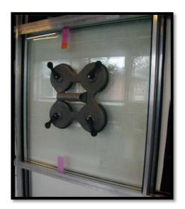
2. Then insert the vertical glazing beads, which must also be hold in place with glazing block wedges. Position the pane correctly and "clamp" it in close contact with the exterior glazing gasket using e.g a glazing shovel.
