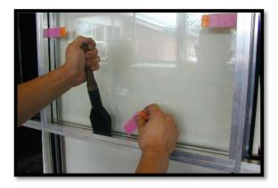
3. The temporary glass fastening shall be maintained until beginning the installation of the internal glazing gasket. However for a maximum of 16 hours due to the risk of thermal breakage of the pane.
