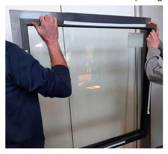
2.2. Pre-set the frame and block it by wedges and mounting spacers in the places of mounting holes. Adjust by wedges and make sure that frame is level in all directions.
