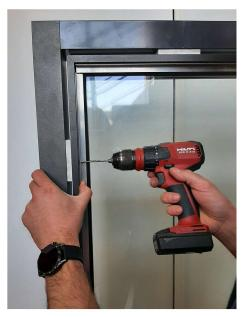
2.7. Install mounting screws. Number of screws correspods to the number of holes in frame
