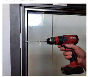
2.8. Check the frame dimensions. If frame has been overtightened, loosen the screw, add spacer and tighten screw.
