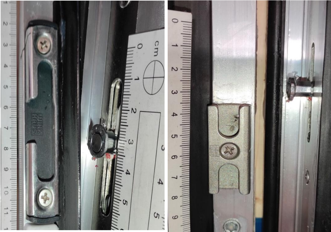
Locking components in frame and sash.
